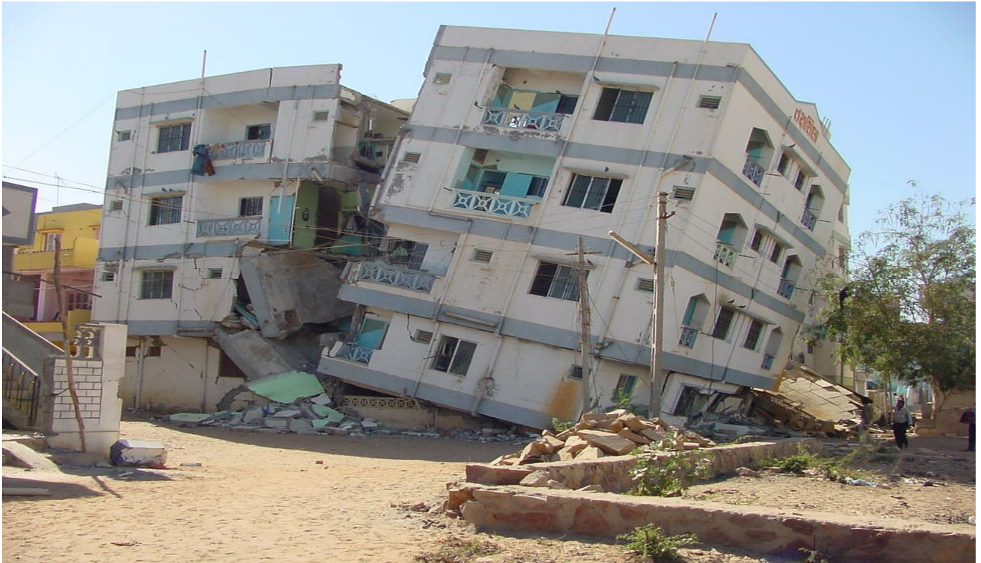
VERTICAL SPLIT BETWEEN TWO BLOCKS (BHUI 2001)
