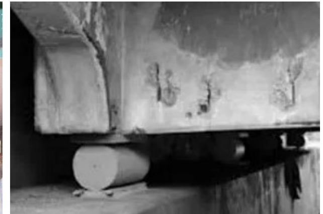
Metallic Rocker-Roller bearings in Seismic zone IV and V
