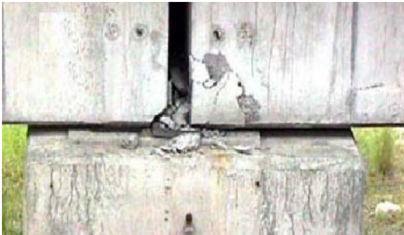
Movement or Pounding of Deck
