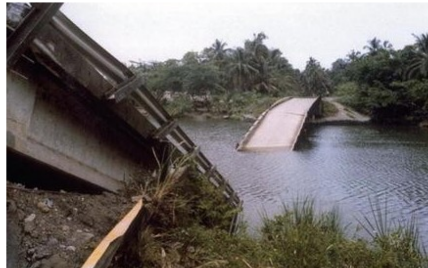
Foundation Failure
