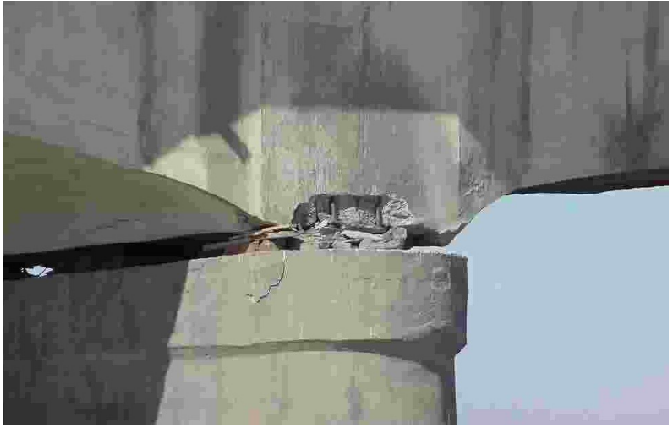
Bearing failure
