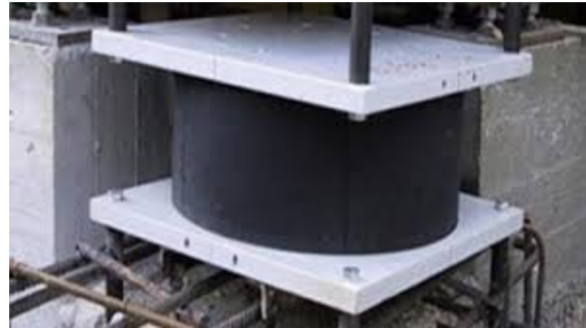
Bearings with high damping characteristics
