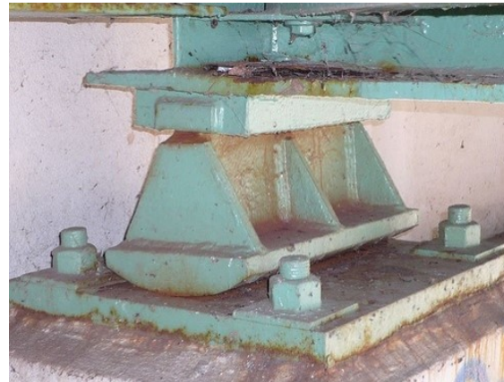
Metallic Rocker-Roller bearings in Seismic zone IV and V
