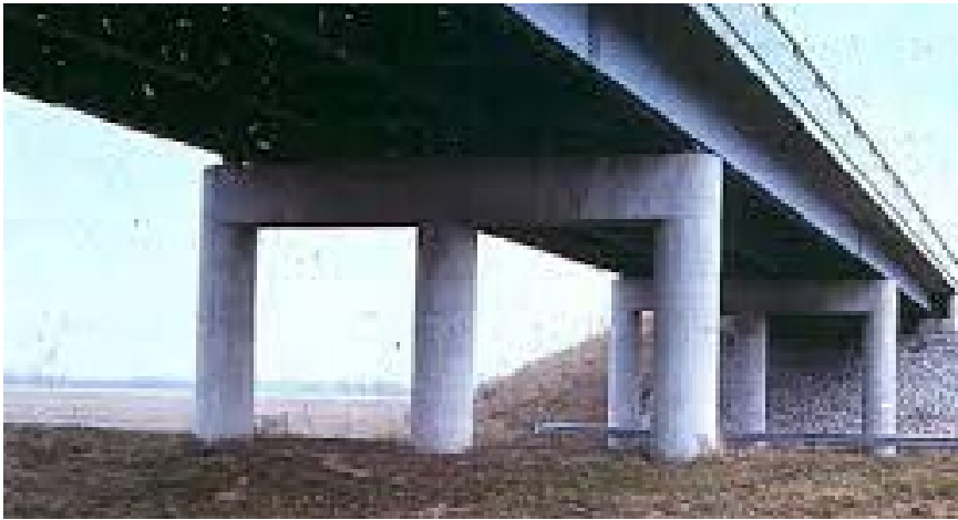
Multiple column substructure
