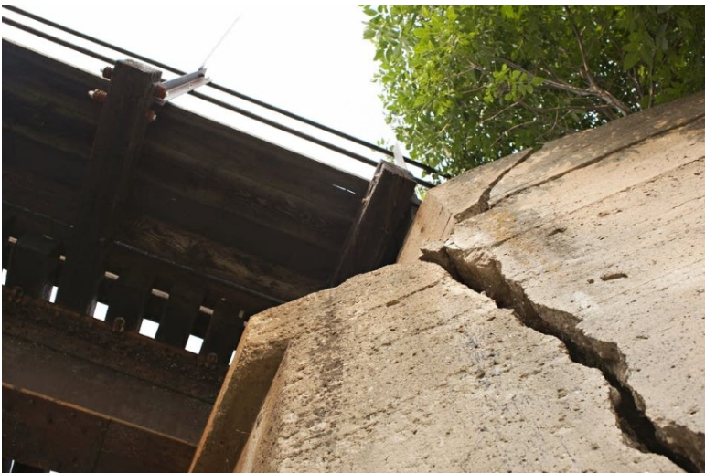
Abutment slumping
